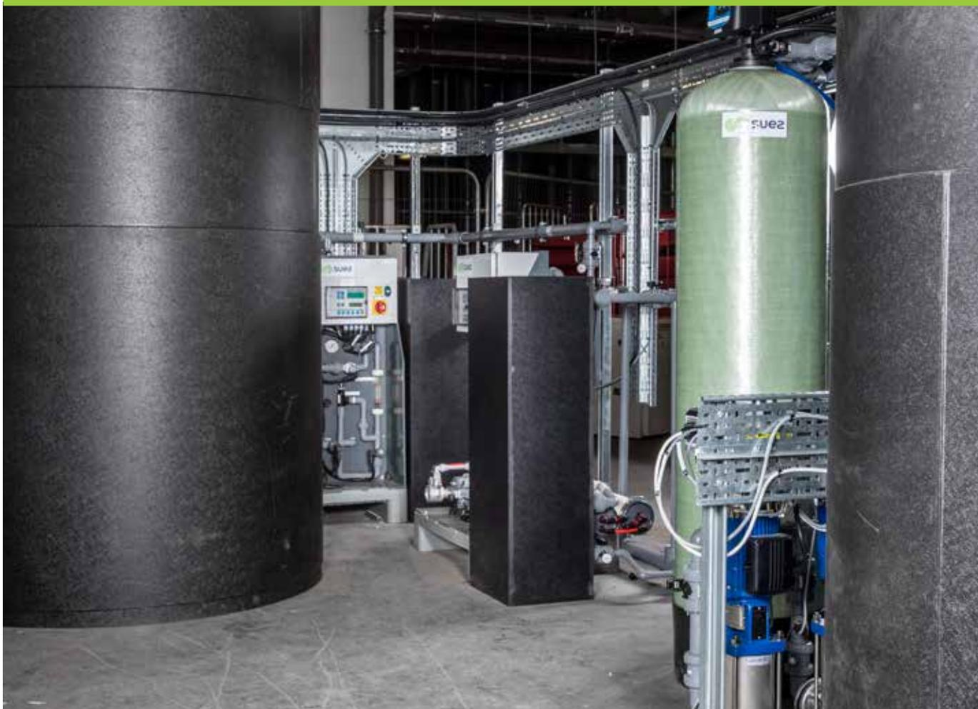
The new Purite system uses an existing raw water supply; due to the nature of the local geology this is already softened, so there is no need to adjust the hardness before the water is subsequently purified. The supply feeds directly into a 2,000l raw water break tank, from where it is pumped through an automatically back-washable carbon filter, via a series of 5-micron filters into two Purite Elite 500 reverse osmosis units, providing duty/standby capability.
